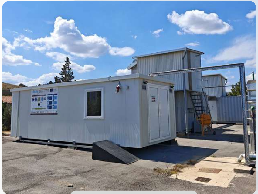
Figure 1. The mobile unit installed at LTCP.
