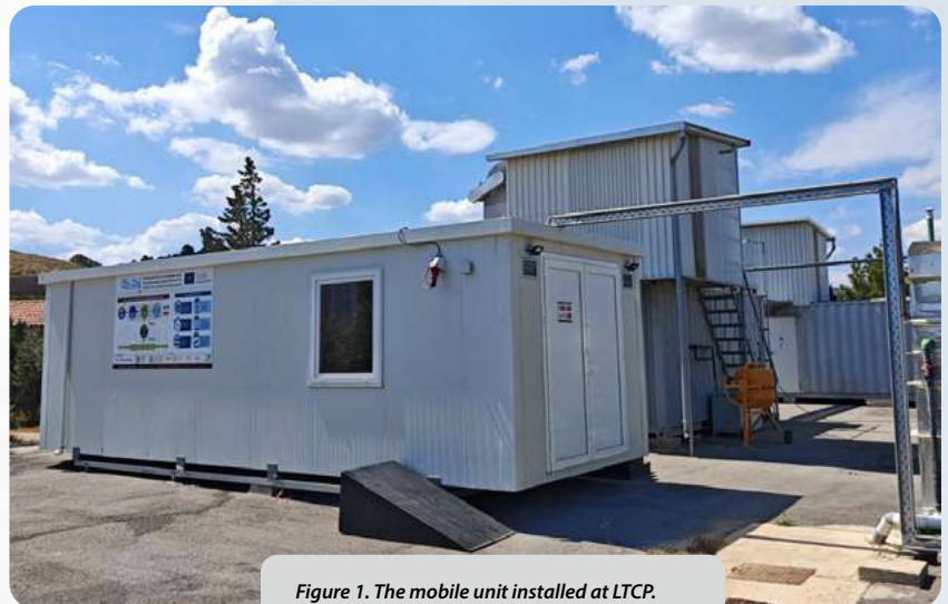
Figure 1. The mobile unit installed at LTCP.
